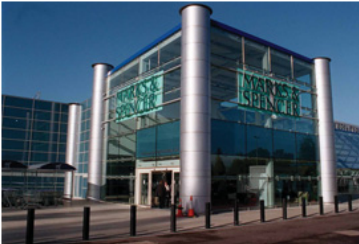
Photo: Marks & Spencer
