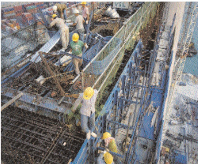
Scientific management on a building site
